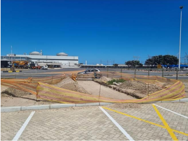
Image 1: Construction of pathway
