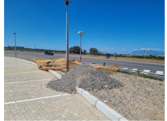
Image 3: Construction materials for the construction of the pathway
