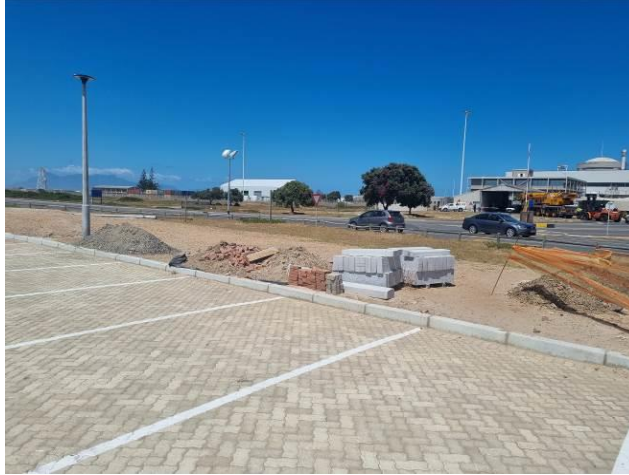
Image 2: Construction materials for the construction of the pathway
